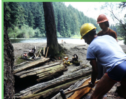
Construction of ACFL signage at Little Cranberry Lake parking lot.
