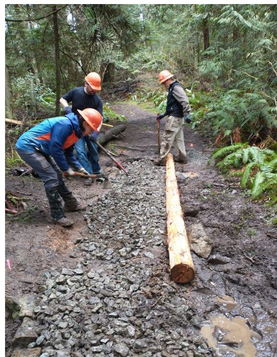
Trail 113 improvements in-progress! Photo courtesy of Washington Trails Association.
